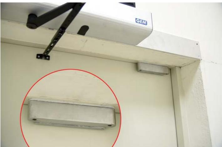
16. It is suggested to install the electromagnetic lock to prevent the door from being opened by force under wind load conditions or access control.
